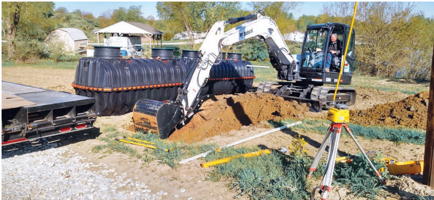
Giant Goose Ranch Excavating to Install IM-Tanks
