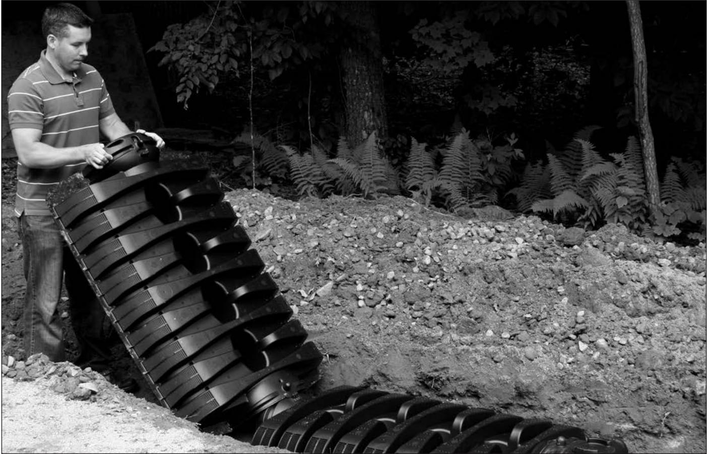
**Note:** When installing in sandy soil conditions, wheeled construction equipment is prohibited over the top of system. Tracked equipment can be used over top of system with a minimum of 6" of soil cover.
