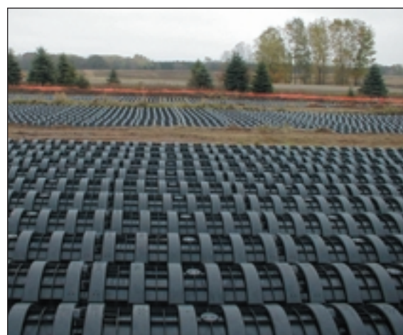
Large community systems using chambers are being designed by engineers due to their large storage capacity.
