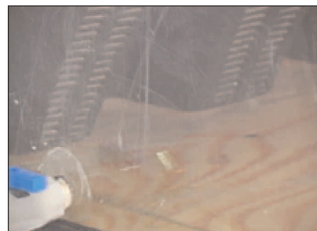
Figure 8: Engineered louvers preventing soil intrusion even after the system has been drained
