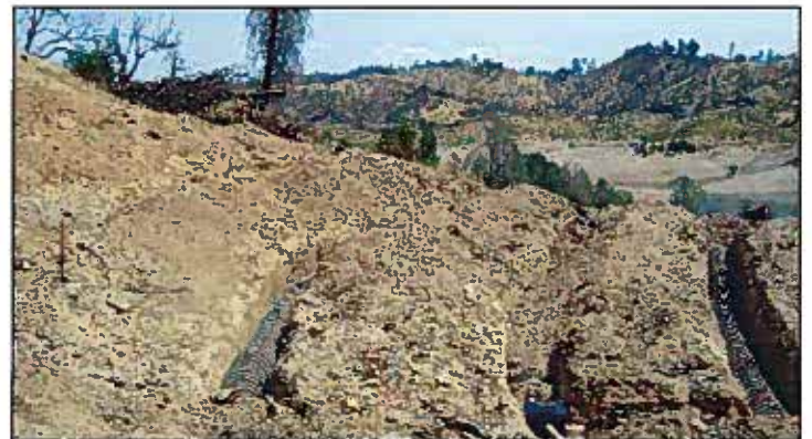
At the Jones Valley Marina, Infiltrator Quick4 Equalizer 36 chambers were chosen for the 1,700 linear foot drainfield due to ease of delivery and installation on sloping terrain.
