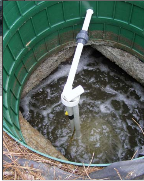
At left, Matt Vinson and Brian Parker prepare to install the air pump and its protective plastic basin. Below, a close-up of the aerobic bacterial generator at work five days after installation.
