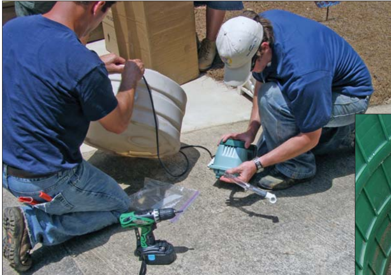
At left, Matt Vinson and Brian Parker prepare to install the air pump and its protective plastic basin. Below, a close-up of the aerobic bacterial generator at work five days after installation.
